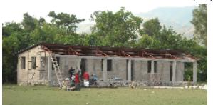
closer to completion. The "stabilized earth block" technology is an environmentally friendly method of building that utilizes locally available materials and provides thermal and seismic advantages over conventional cement block construction. In December the building is scheduled for completion when Jeff Rottler, from the **Tierra y Cal Institute** in Mexico, will train the local construction team in techniques of natural earth plastering and flooring.
